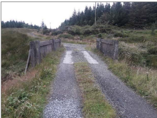
Figure 24 - Bridge 6 on access to Windfarm Site boundary
