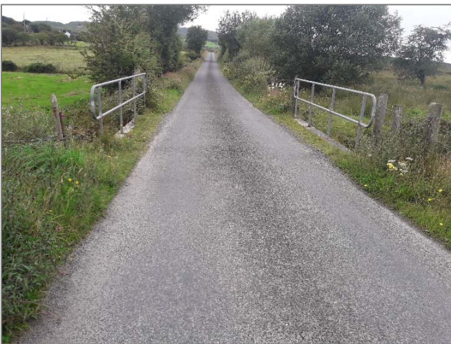
Figure 16 - Bridge 2 within L-7211-2
