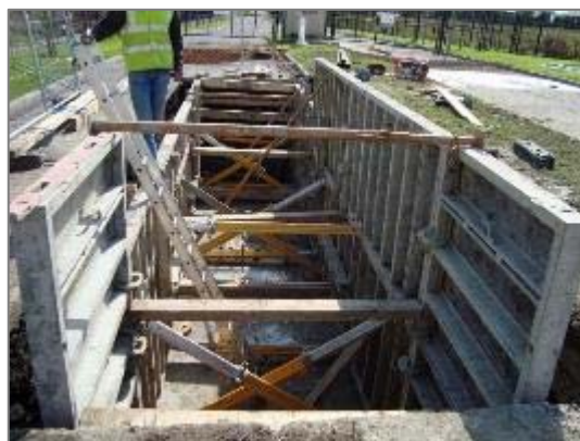
Figure 7- Typical joint bay under construction (in-situ)
