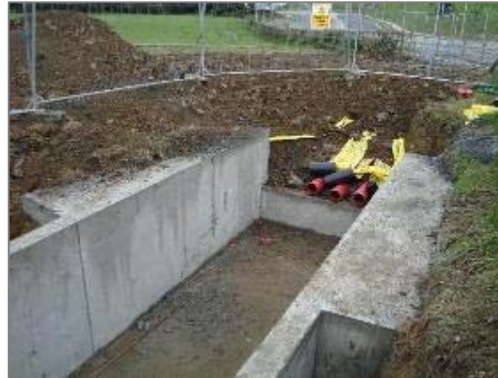
Figure 8 - Completed joint bay prior to cable installation (in-situ)
