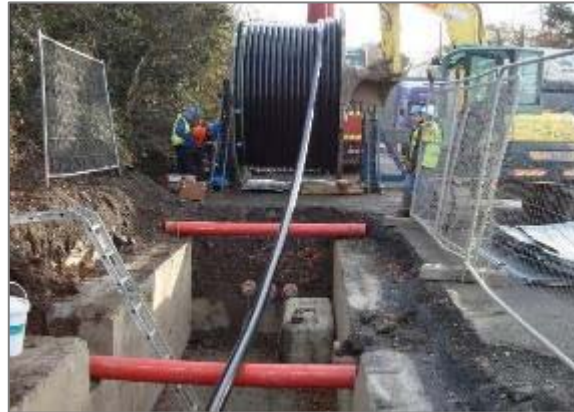
Figure 10 - HV cable pulling procedure (Typical drum set-up)
