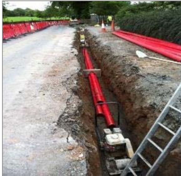
Figure 2 - Typical 110kV Underground Duct Installation
