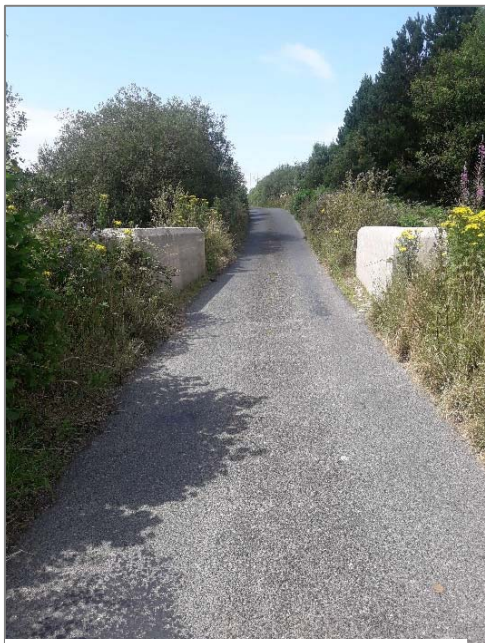
Figure 14 - Bridge 1 Location within L-7211-2
