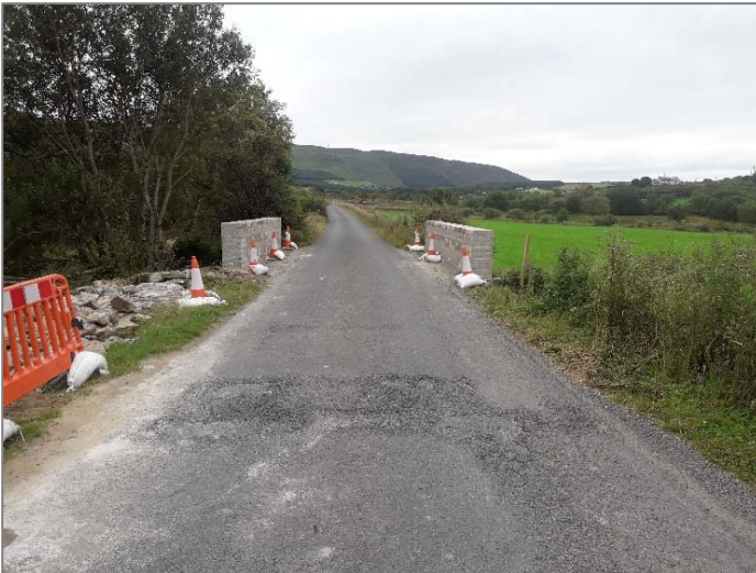
Figure 18 - Bridge 3 within the L-7261-1
