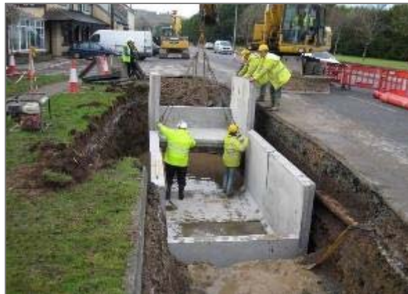
Figure 9 - Typical joint bay under construction (pre-cast)
