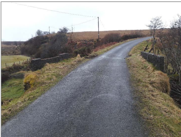
Figure 23 - Bridge 5 within the L-7241-2
