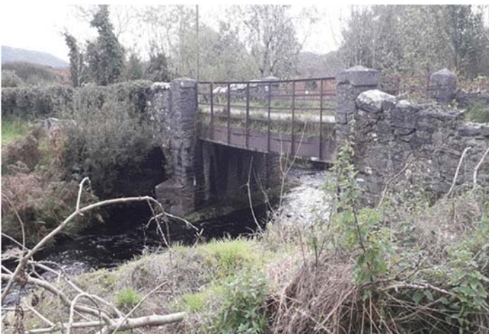
Figure 20 - Bridge 4 within the L-1781-3
